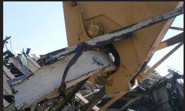
▲▲▲▲▲▲▲▲▲▲▲▲▲▲▲▲ Cold Cutting of Industrial Plants Using Specialised Hydraulic Shears
