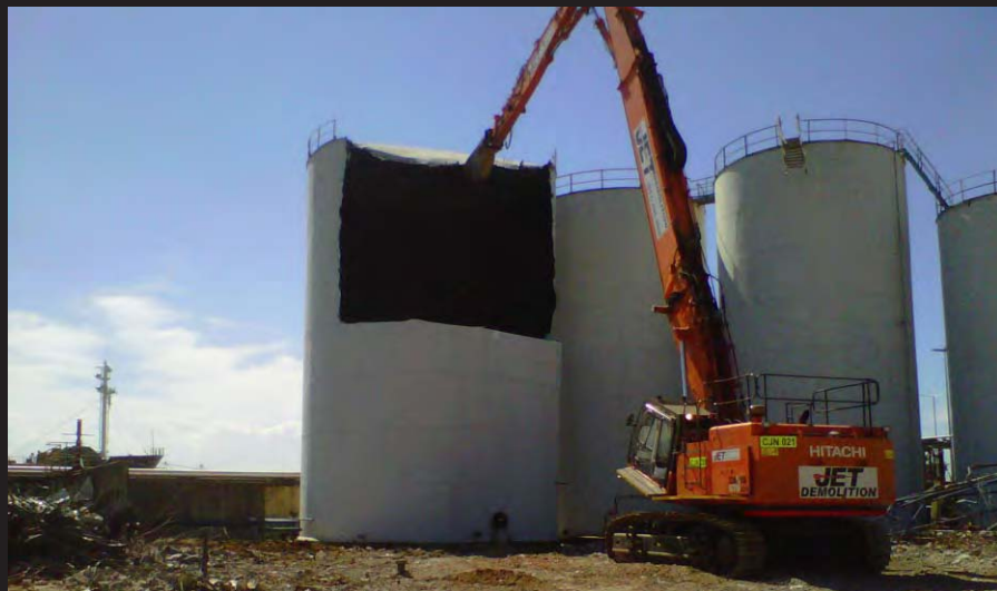
▲▲▲▲▲▲▲▲▲▲▲▲▲▲▲▲ Demolition of Petrochemical Tank Using Specialised Hydraulic Shears
