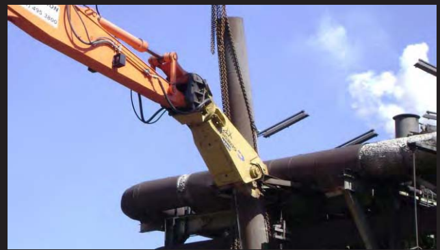
▲▲▲▲▲▲▲▲▲▲▲▲▲▲▲▲ 80 Tonne Demolition Excavator with a Large Specialised Demolition Shear
