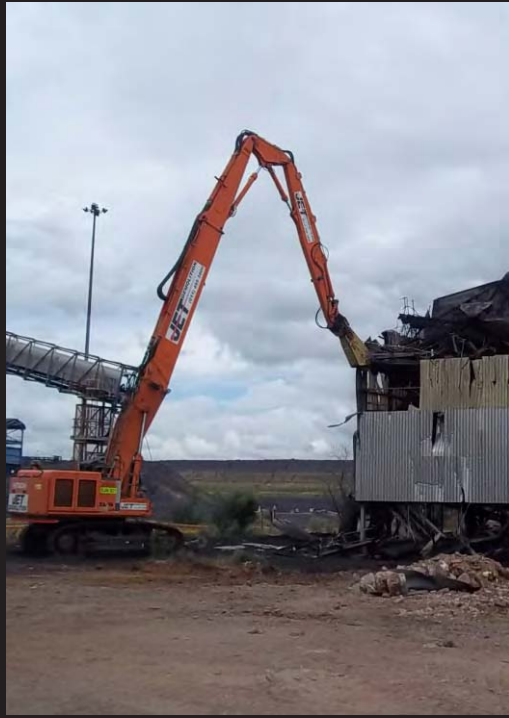
▲▲▲▲▲▲▲▲▲▲▲▲▲▲▲▲ Mechanical Demolition of PSS Plant
