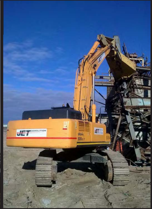
▲▲▲▲▲▲▲▲▲▲▲▲▲▲▲▲ Demolition of Heavy Steel Crusher Structure by a Large Hydraulic Shear
