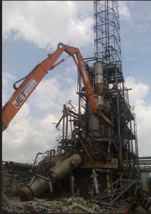
▲▲▲▲▲▲▲▲▲▲▲▲▲▲▲▲ Rapid Demolition of Acid Plant by High Reach Excavator
