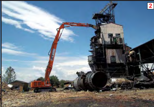
Safe Top-Down Demolition of Chimney
