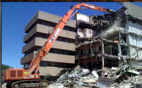
Controlled Mechanical Demolition of Concrete and Steel Structures
