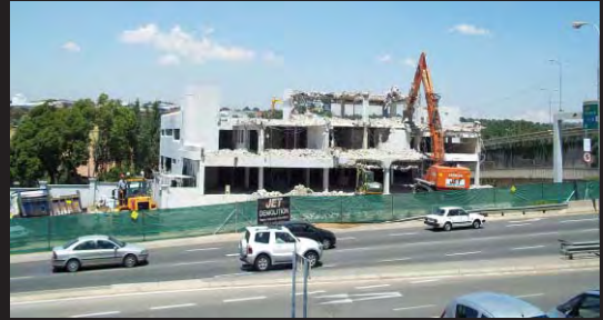
Controlled Partial Demolition for Refurbishment
