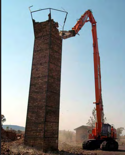
Safe Top-Down Demolition of Chimney
