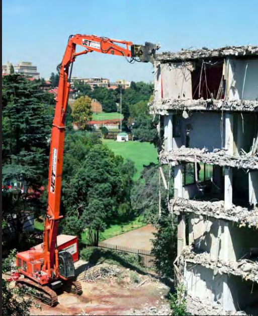
Controlled Demolition of Building Containing Fully Operational Municipal Substation
