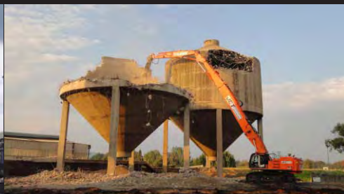
Demolition of 3 Gas Producers Located 1 m from a Storage Building Which Remained
