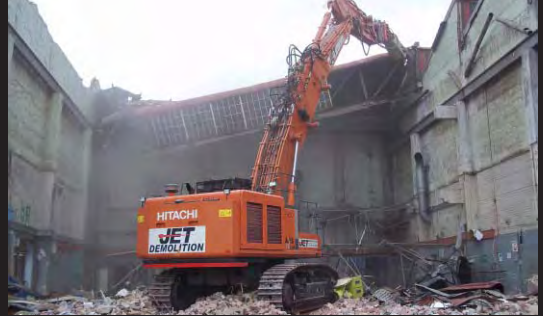
Controlled Demolition of Steel & Concrete Structure Adjacent to Operating Gas Plant
