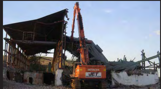
High Reach Excavator Demolishing Mine Shaft Winder House
