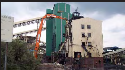
Demolition of 3 Gas Producers Located 1 m from a Storage Building Which Remained
