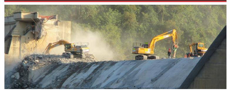
REHABILITATION OF DAM WALLS USUALLY REQUIRES DEMOLITION OF REDUNDANT PORTIONS OF MONOLITHIC BLOCKS. JUDICIOUS SELECTION OF DEMOLITION METHODS AND THEIR APPLICATION TECHNIQUES ARE VITAL TO A CONTROLLED AND PRODUCTIVE PROJECT.
